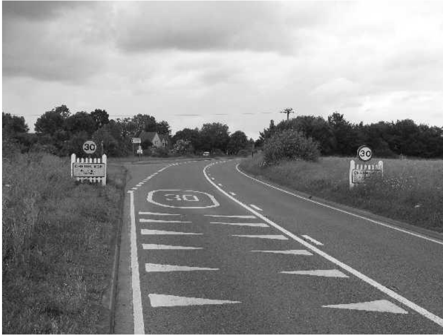
Figure 6.5. Example of a village entry gateway treatment
